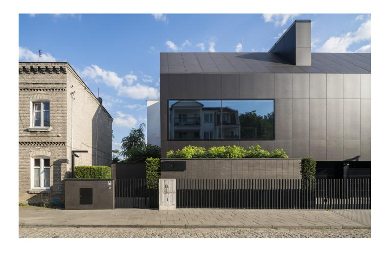
Herba House has two distinct faces, closed to the street and open to the river. The "house" to the street facing northward is clad in black Swisspearl panels, while the southern part of the house consist of terraces that open out onto the riverside and cascade down the slope.
