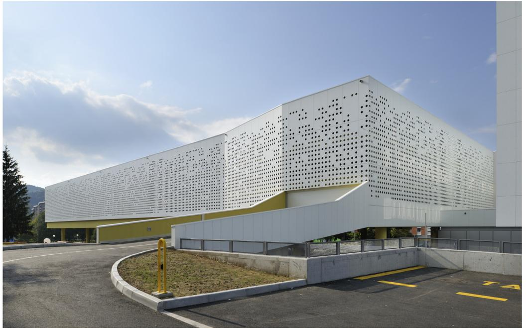
This building in Velenje is a spacious bus station at ground level and offices and a parking garage on the upper floors. The superstructure is notable for its extensive white Swisspearl panelling that serves to unify the different sections. The irregular pattern of perforations creates a distinctive day and night contrast.
