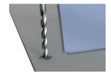
If not using Swisspearl Facade Wing Screws, the boards should be pre-drilled with an appropriate fibre cement drill bit. Dust from cutting or drilling must be removed with a brush or a fiber cloth immediately after the work has been completed, otherwise it can mark the surface of the boards.
