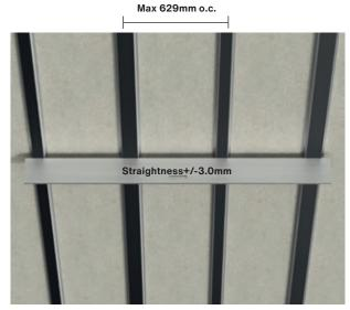
Straightness of substructure
