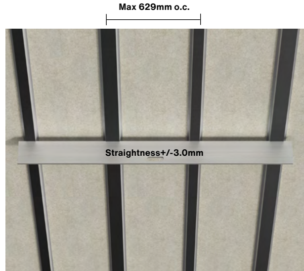
Straightness of substructure
