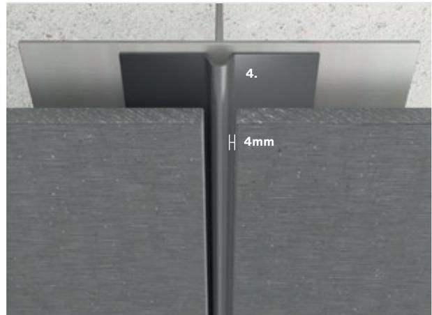
Swisspearl Caulking Profile can be used in both vertical and horizontal joints. It is not mandatory to use Swisspearl Caulking Profile, but it provides excellent joint solutions. The profile is installed in the same way as Swisspearl External Corner.
