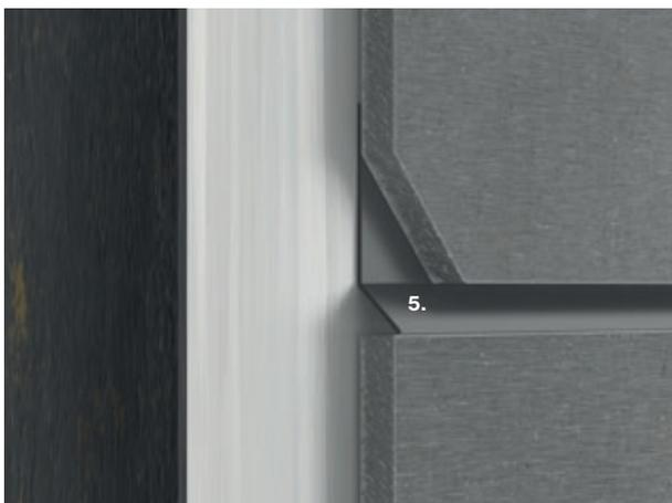
The Horizontal L Profile used for horizontal joints should be cut in the same length as the width of the facade board.
