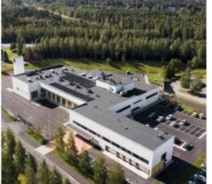
We ended up using fibre cement boards, which made the facade more welcoming and pleasant to touch. It also makes the surface more lively. Swisspearl's through coloured fibre cement boards are very durable and weather resistant, and it is easy to change the boards when needed. The facade is durable and easy to maintain, which also makes it life cycle economic and ecological.
