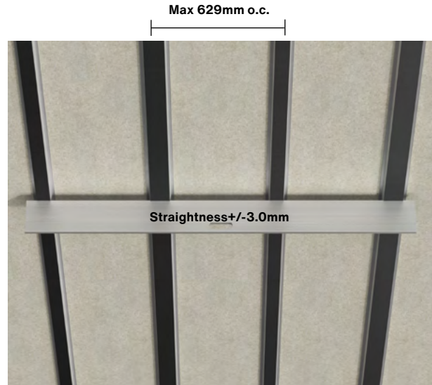
Straightness of substructure
