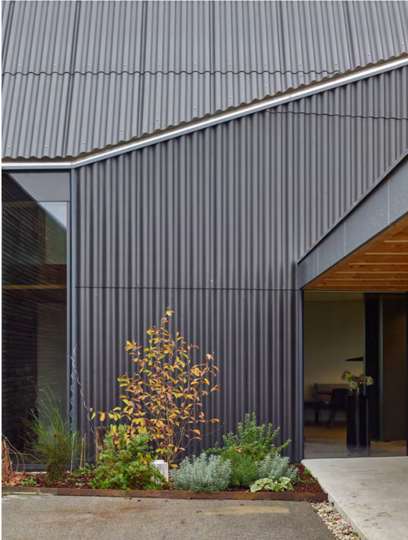
Residential BK, Lambach, Austria. Architect: Arch. DI Bettina Brunner-Krenn, Lambach, Austria. Photographer: Kurt Hoerbst, Rainbach, Austria.
