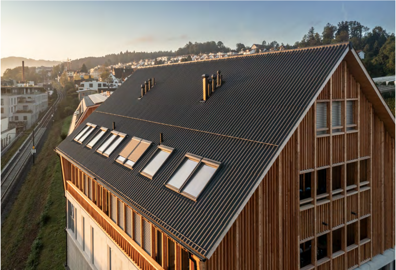
Student Residence, Wädenswil, Switzerland. Architect: Hotz Partner AG SIA, Zurich, Switzerland. Photographer: Meraner & Hauser OHG/SNC, Bolzano, Italy.
