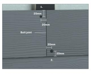
When butt jointing, make sure planks are loosely butt jointed.
