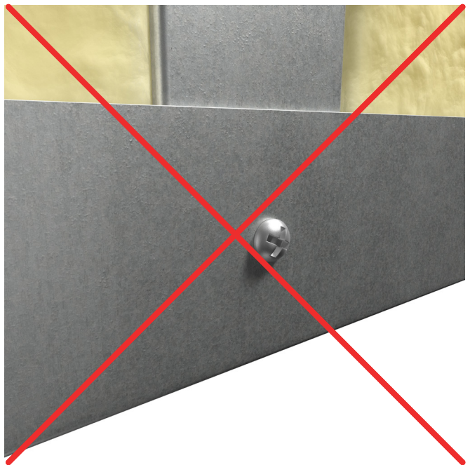
The use of screws with excessively large heads must be avoided.
