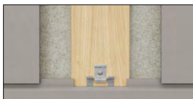
Photo 2 Clips Swisspearl Plank Connect
