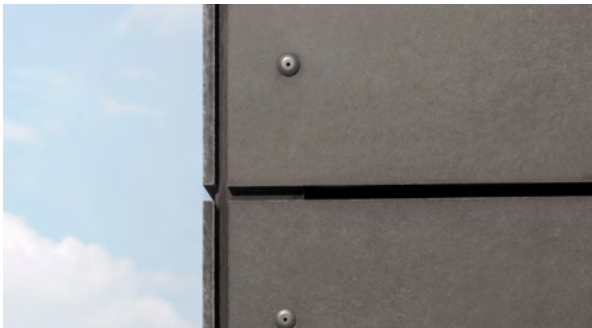
Visible mounting of the fiber cement panels with colored rivets
