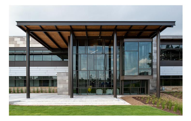
Neptune Office Building is articulated in long, extended parallel lines of layered materials: stone, glazing, Swisspearl panels, and steel flashing in tightly packed, overlapping panels. Interlocking forms protrude from the facade envelope covered by the timber-clad eaves overhang that protects the upper floor outdoor balcony.
