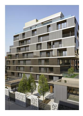
The brief for this project in Milan called for the urban renewal of the area and the renovation and conversion of the building for residential use. Sliding, screen-printed glass panels and black Swisspearl panels on the facades create a dynamic pattern of shifting planes held between the horizontal concrete floor slabs.
